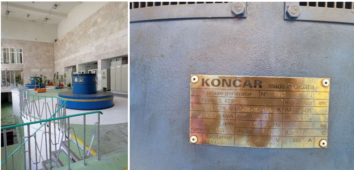
Source: Fichtner, taken during site visits in 2022 Figure 33: Generators in Globocica and generator nameplate
