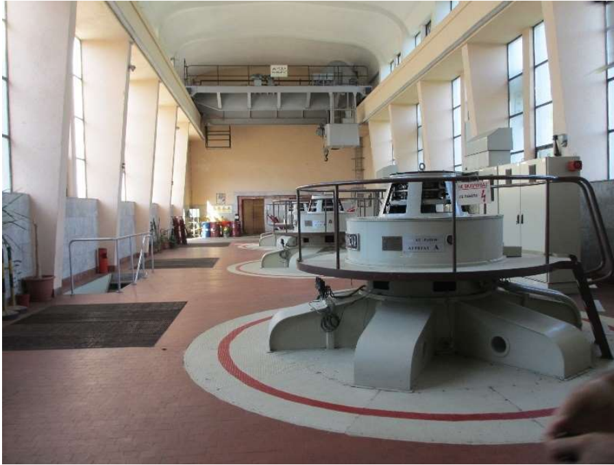
Figure 28: Generators in HPP Raven
