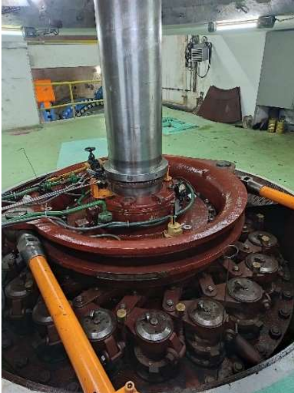
Figure 34: Wicket gates of Francis turbine
