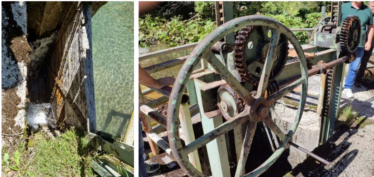
Figure 21: Stirovica gates and operational mechanism
