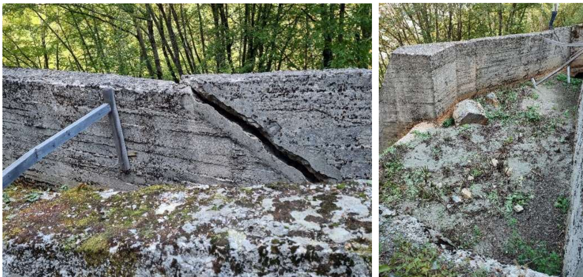
Figure 27: Damaged sedimentation tank
